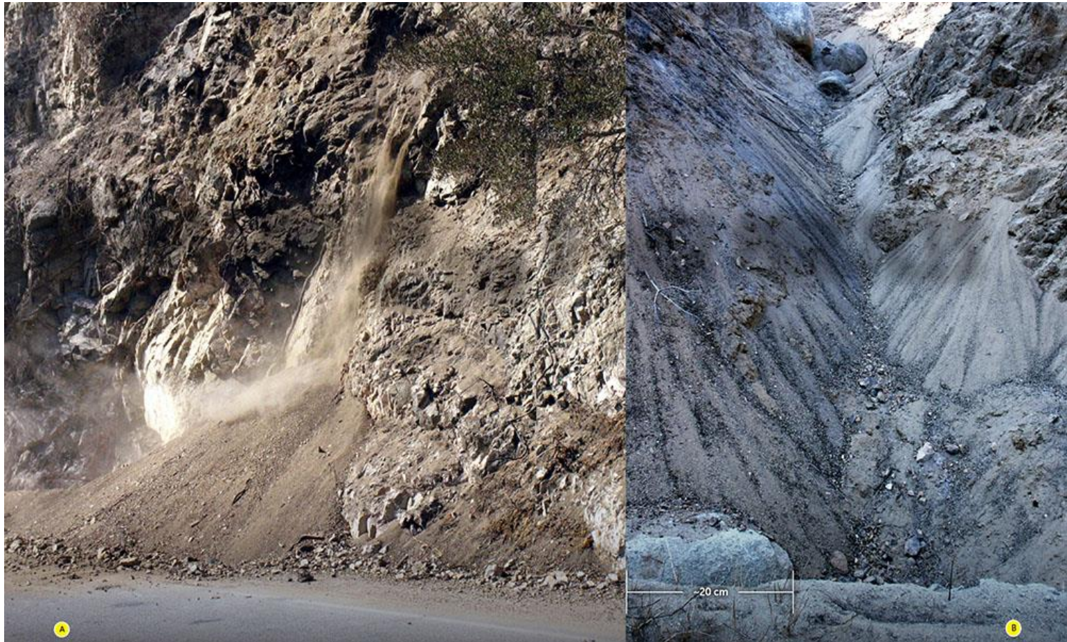
(Left) Talus cone of active ravel onto S.R. 2, LA County, during 2009 Station Fire, and (Right) accumulated ravel following the 2003 Cedar Fire in San Diego (Keaton et al. 2019)
